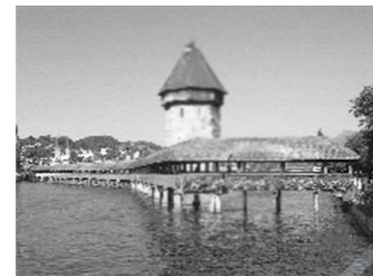
The Chapel Bridge
