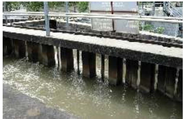
Fig. 18.4 Grit and sand removal tank
