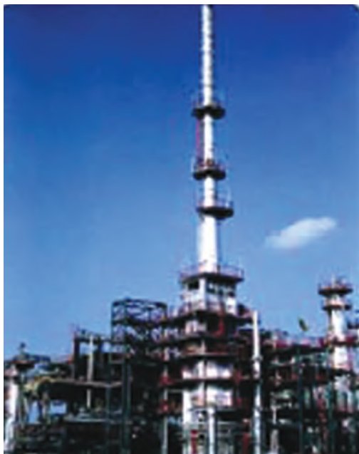
Fig. 5.5: A petroleum refinery
