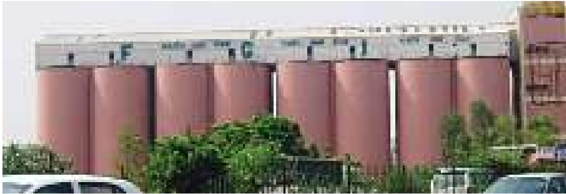
Fig. 1.10 (a) : Silos for storage of grains
