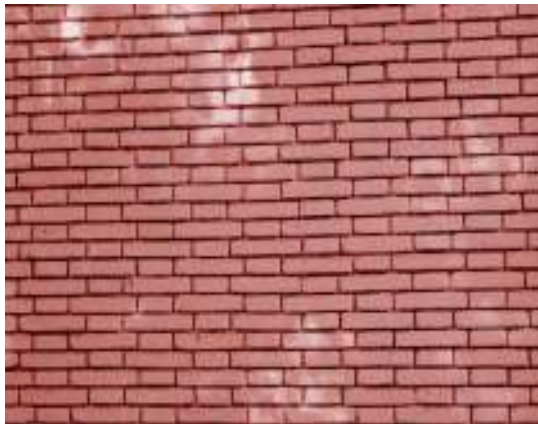
(a) Brick wall
