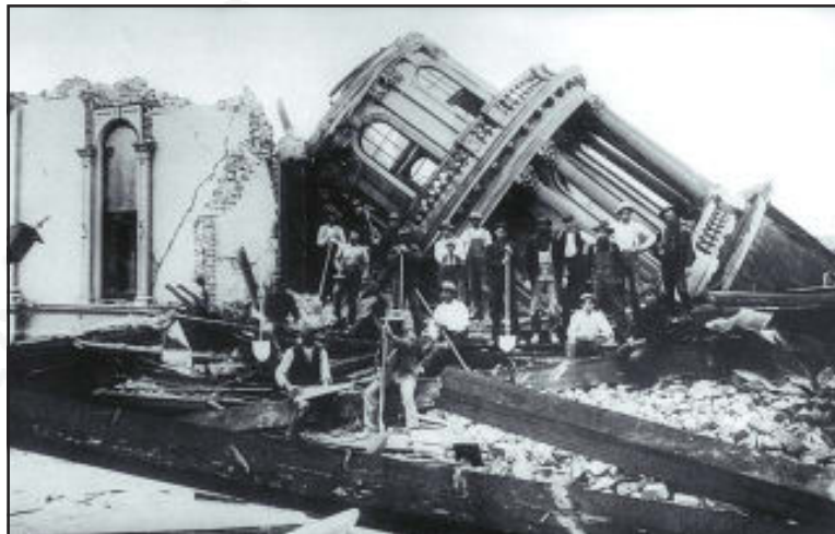
Fig. 2. Buildings destroyed by an earthquake.
