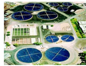
Fig: An aerial View of a Sewage plant
